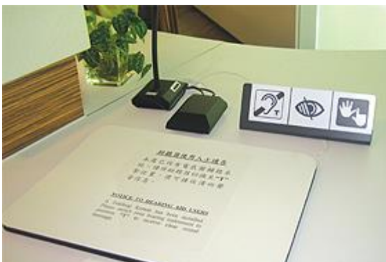
Induction loop system - an assistive listening tool for hearing impaired persons.
