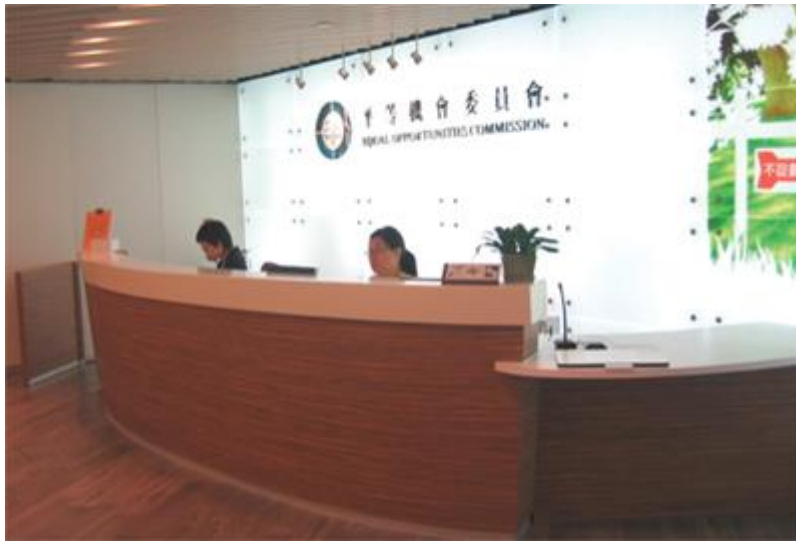
Low level counter top for wheelchair users.
